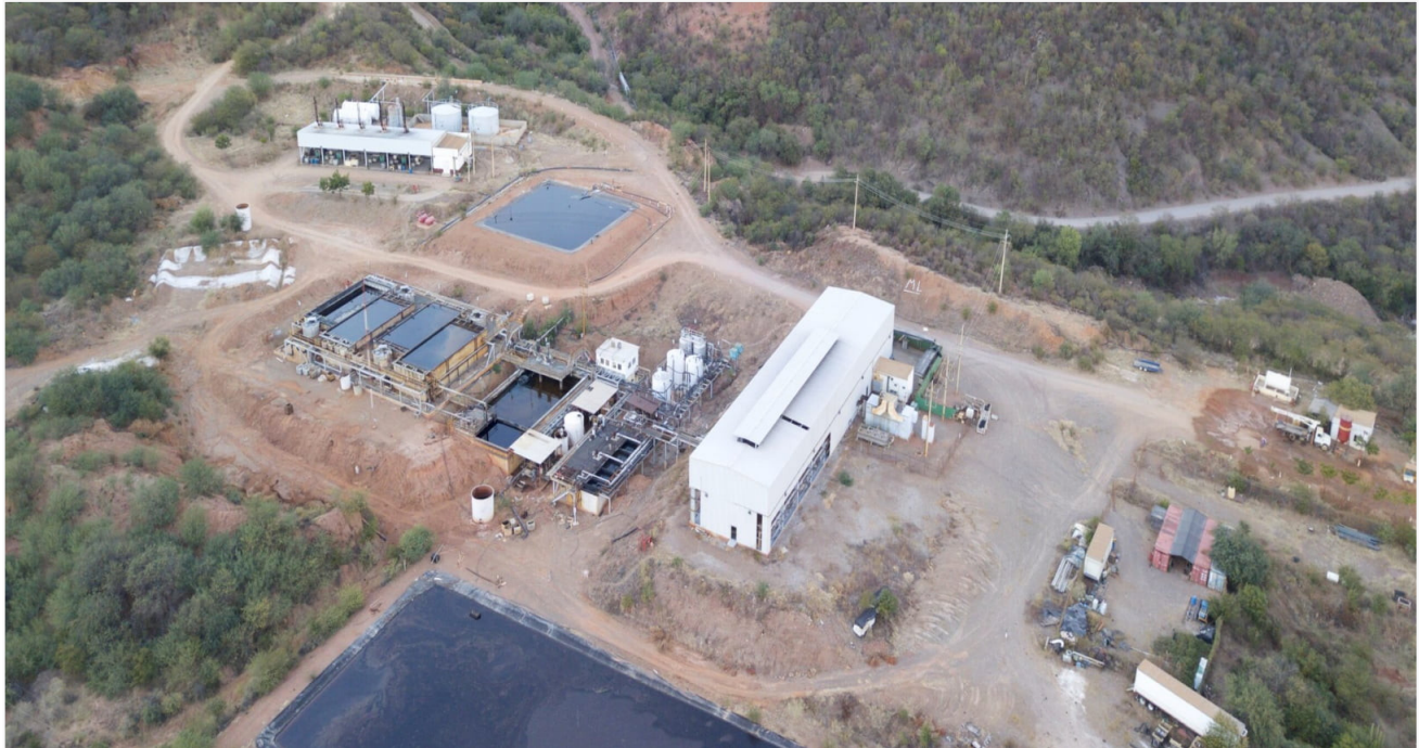
Figure 3: On site processing facilities inclusive of a carbon-in-column plant
